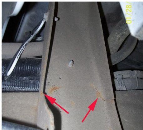
Figure 1: Example of a front mount bracket cracking as a result of not all mounting locations being utilized
