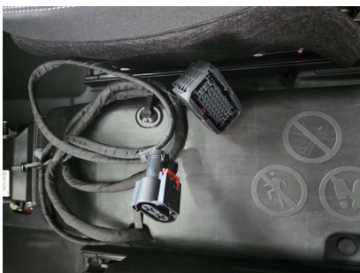
Located under console
